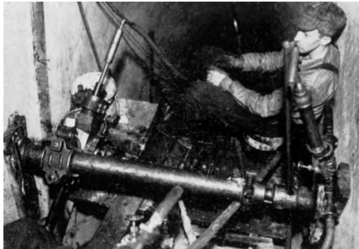
**Figure 5. Cramped working spaces typified the 9-year program of extending the grout curtain, from the dam's lowest centerline gallery between 1938 and 1947 (USBR).**
