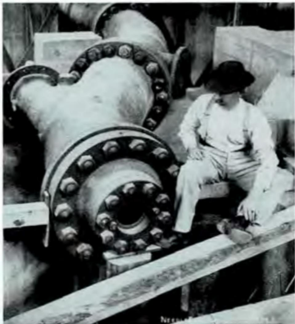
At the bottom end of the pipelines from the reservoir high above lies this complex casting, the "needle-valve housing." Inside this pipe, a long, slender "needle valve" travels back and forth to regulate the flow of water onto the water wheel, thus regulating the electrical output of the generators. This photo of one of the four needle valve housings in Powerhouse No. 1 gives an idea of the small hole through which the water must flow.
