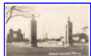
Posey Tube Oakland Side
