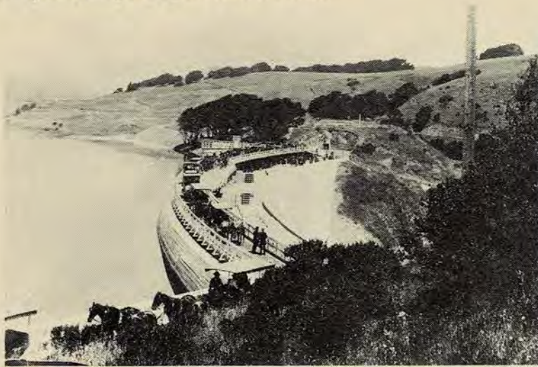
In 1896, members attending the American Society of Civil Engineers convention visited Crystal Springs Dam, a pleasant day's outing by carriage.
