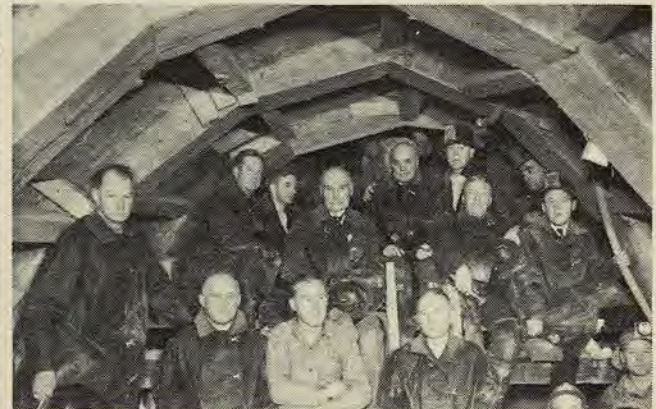
Tiny Niles Dam (top), shown under construction in 1897, is the first point of diversion for Alameda Creek water. (Above) A tired looking Michael O'Shaughnessy (second row, fourth from left) attended the holing through of the Coast Range Tunnel on January 5, 1934.
