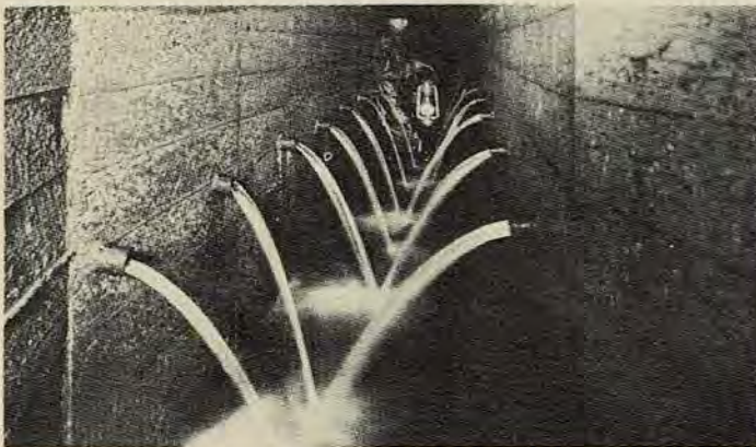
Graceful Sunol Water Temple (top) marks the location of the underground percolation galleries (above) which are the key to gathering water from the Sunol Valley.
