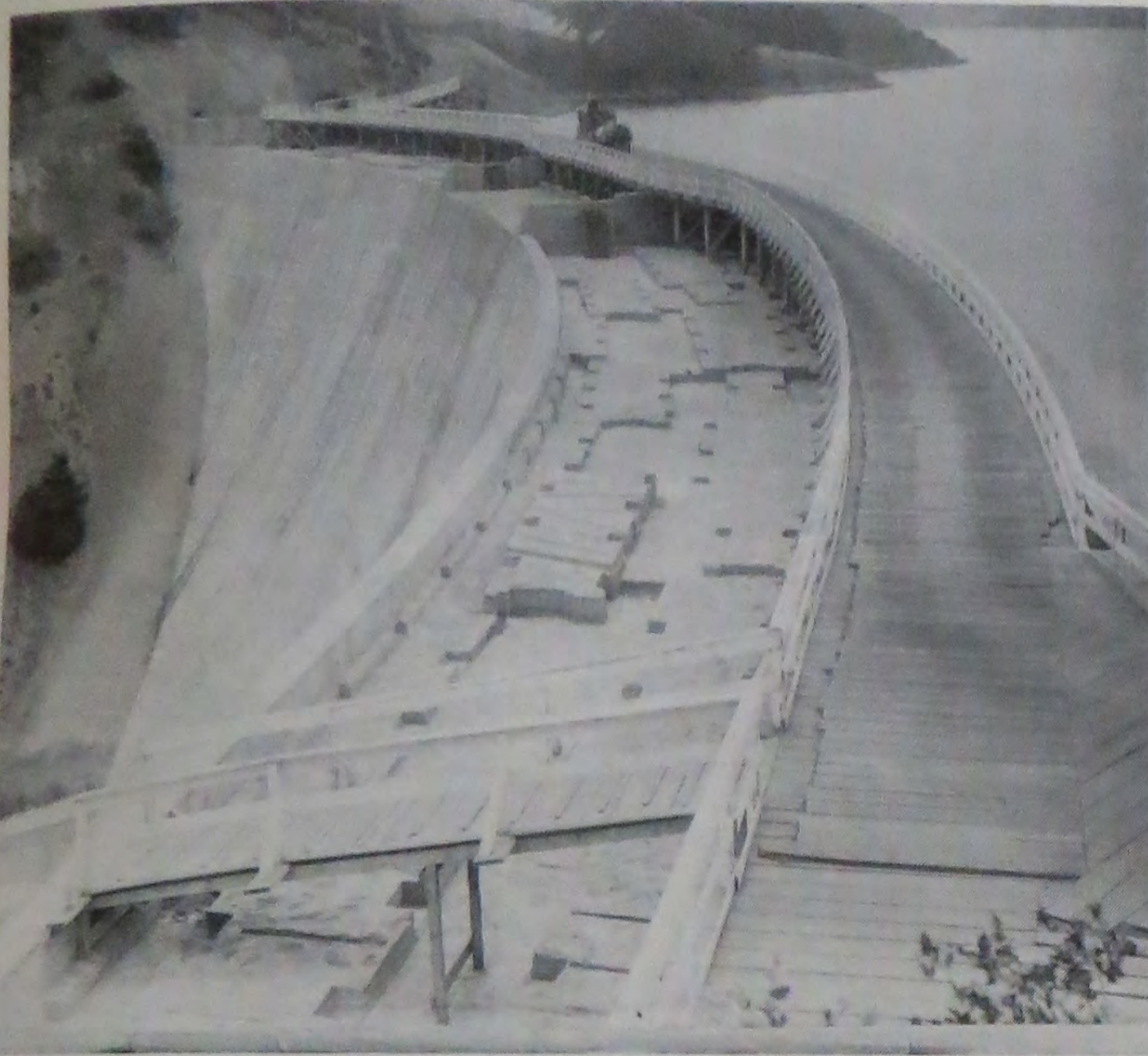
Figure 2-4 Photo of crest—Lower Crystal Springs Dam
