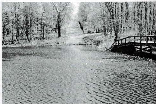
Fig. 2. Site of one of the 23 incline planes on the Morris Canal (with slack-water towpath bridge below) that were required to overcome the cumulative rise and fall of 1,674 ft as the canal crossed New Jersey. The Morris Canal was designated a NHCEL in 1980.
