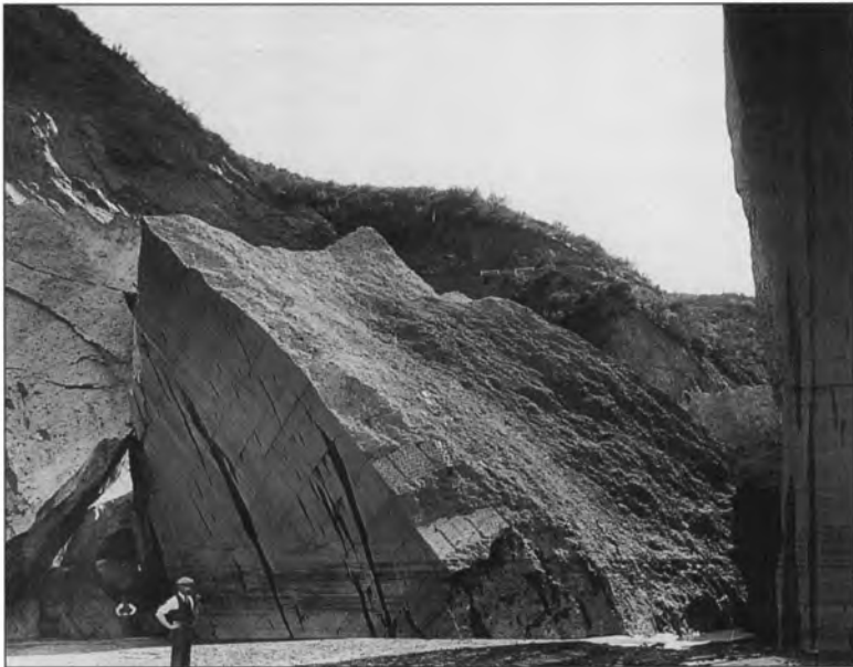
Figure 31 (lower) - Ground view looking at upstream face of Block 2 and east edge of Block 1, showing silt scour lines approximately 15 feet above the infilled reservoir floor. These water lines suggest that Blocks 2/3/4 toppled over late in the flood sequence, when only 20 to 25 feet of water remained in the reservoir. Huber Collection, University of California Water Resources Center Archives.
