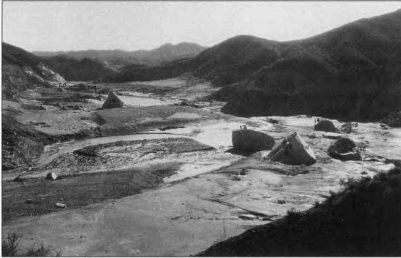
Figure 29 (upper) - Ground view of Blocks 13, 14 and 11 (left to right), as seen from across the canyon 400 yards downstream of the dam the morning after the failure. Note the enormous bank of schist silt and detritus upon which the blocks were deposited. Photo from University of California Water Resources Center Archives.
