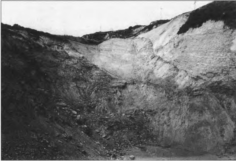
Figure 16 (upper) - View looking uphill into the evacuation scar of the 1928 east abutment slide, as seen from the floor of the canyon, just downstream of the dam's former position. This photo shows the guardrail of San Francisquito Canyon road parallel to the slide's west headscarp, thereby fixing its relative vertical position (as shown on Figure 17). Photo by permission of Ventura County Museum of History & Art.
