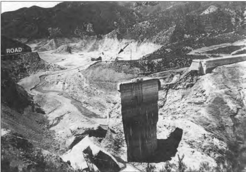
Figure 28 - Overview of the flood's aftermath, immediately downstream of the dam. The flood wave scoured the canyon's slopes to a maximum depth of 120 feet above the stream level. Edison's Bore line crossed the channel, but was situated above the maximum scour line (arrow). San Francisquito Canyon road began climbing east wall of the canyon, at upper left. Photo from University of California Water Resources Center Archives.
