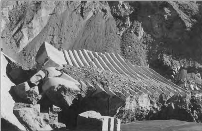
Figure 22 (lower) - Close-up of Blocks 5 and 6, as seen after the failure. The two lowermost steps of Block 1 remained intact. Note the accumulation of schist detritus upon Block 5, about 25 to 30 feet above the creek bed.
