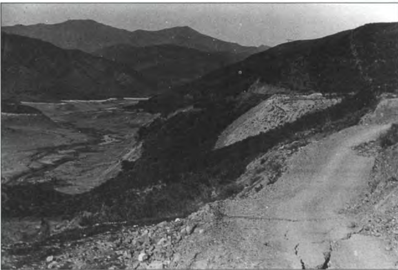
Figure 16 (lower) - View looking up-canyon from the highline, or surge chamber road, immediately above the east abutment slide headscarp (position "A" in lower portion Figure 15), a few days after the failure. Retrogressive tension scarps reached 200 feet uphill of the slide, dropping this upper road by about 10 feet. Note the tandem poles of the Edison Borel power line, well above the level of the reservoir. In this area the highline road approximates the headscarp of the ancient landslide complex shown in the lower half of Figure 1.
