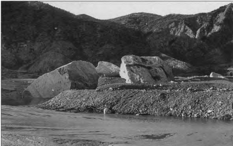
Figure 29 (lower) - Portion of panorama of displaced dam blocks, looking downstream from a position about 300 yards downstream of the dam. Block designations are those of the Governor's Board of Inquiry (Figure 9). Photo from Lippincott Collection, University of California Water Resources Center Archives.
