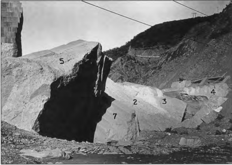
Figure 31 (upper) - Ground view looking upstream on east side of Block 1 at Blocks 5, 7, 2, 3 and 4. The scour hole containing Blocks 2 and 3 must be approaching 60 feet deep in order to have accounted for their buried mass. Huber Collection, University of California Water Resources Center Archives.
