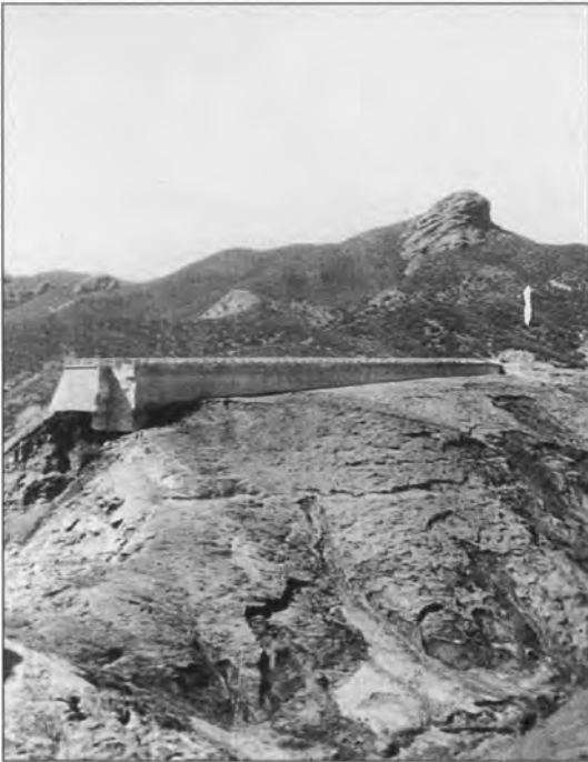
Figure 7 (lower) - Approximately the same view, as seen the following day, after the dam failed, leaving the west dike in place. Water had been leaking from beneath this dike the previous day. Note the widespread occurrence of shallow earthflows on the Sespe slope, likely due to rapid drawdown-induced pore pressure differential as the reservoir emptied in less than an hour. Photo by permission of Ventura County Museum of History & Art.
