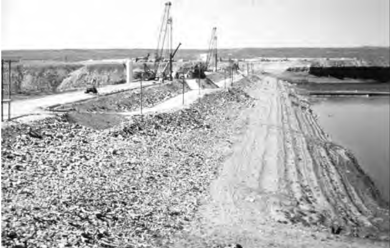
Figure 19 - Fontenelle Dam - Diaphragm Wall Construction
