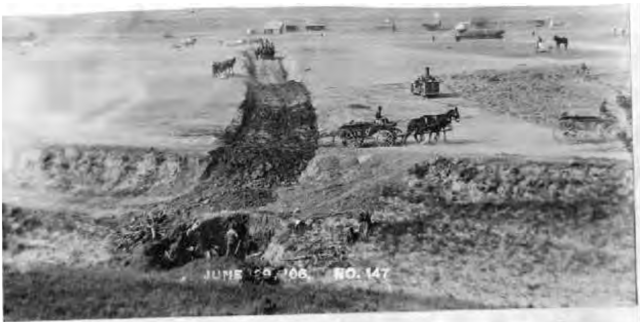
Figure 6 - Belle Fourche Dam - Cutoff Trench Construction
