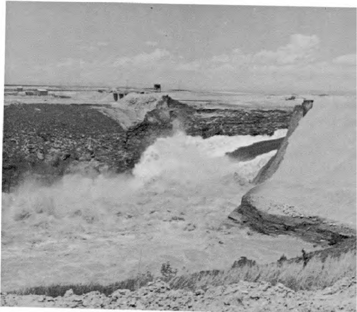
Figure 17 - Teton Dam - Dam Completely Breached
