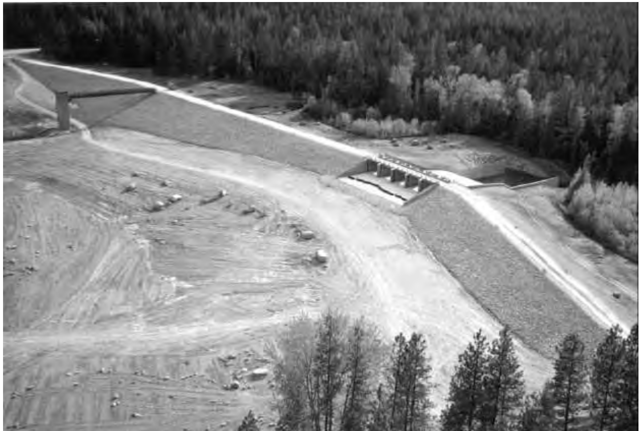
Figure 22 - McDonald Dam - New Dam in 2000
