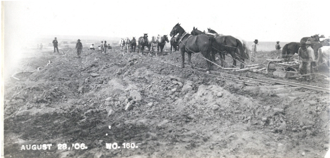
Figure 8 - Belle Fourche Dam - Embankment Fill Construction
