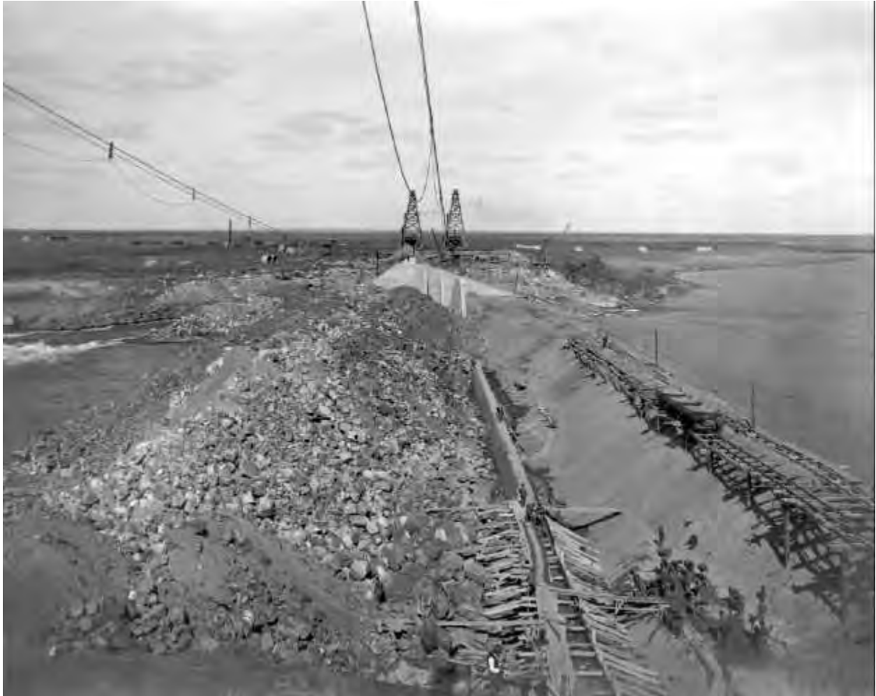
Figure 4 - Minidoka Dam Construction
