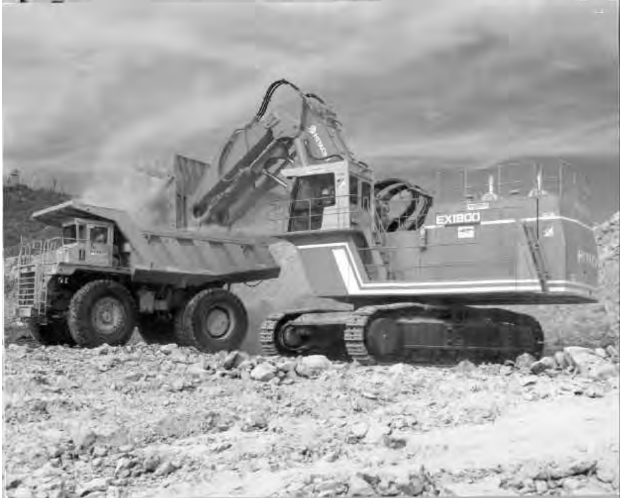
Figure 24 - New Waddell Dam - Construction Equipment
