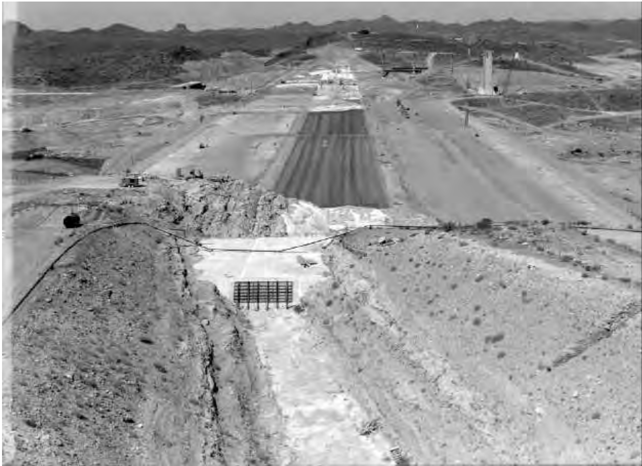
Figure 23 - New Waddell Dam Construction
