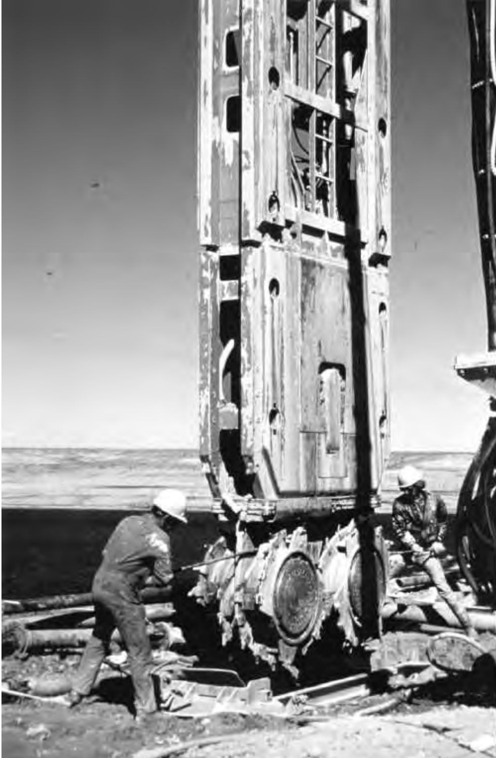
Figure 20 - Fontenelle Dam - Diaphragm Wall - Hydromill Rock Excavator
