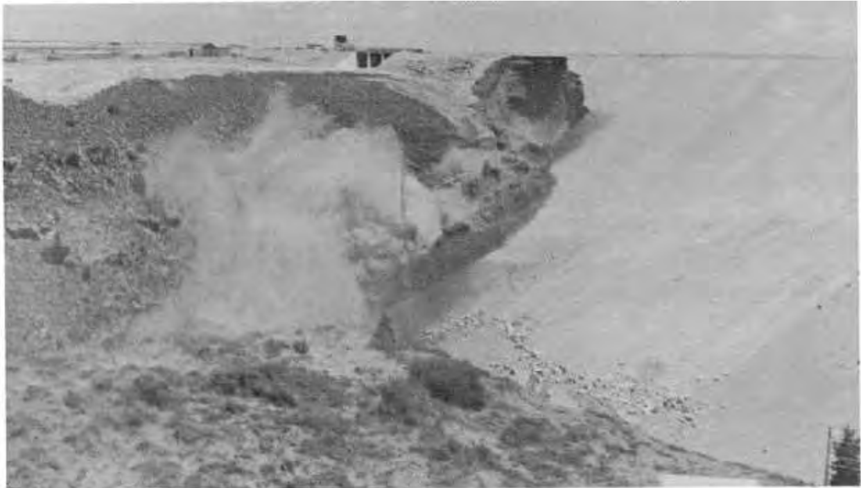
Figure 27.—Dam crest breaching 11:55 a.m., June 5, 1976.
