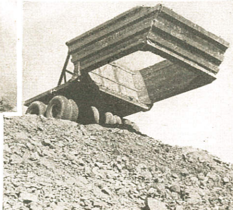
The empty "buggy" after its load has fallen through the open bottom onto the side walls of the canal
