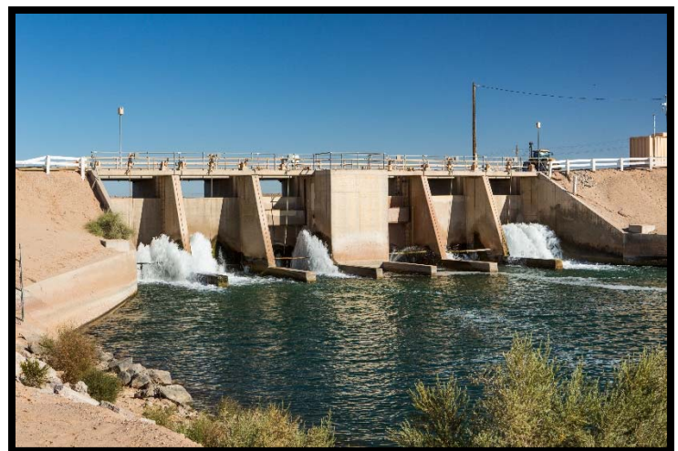
Based on innovative design features and the ability to foresee future environmental impacts, the All American Canal System has withstood the test of time
