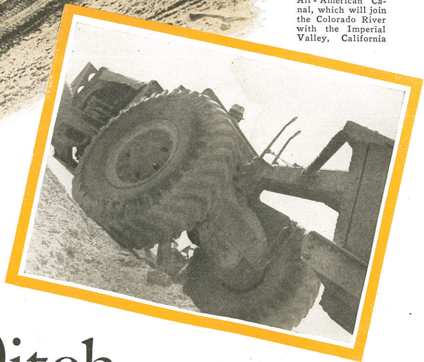
The big balloon tires on this tractor keep it from sinking into the sand as it pulls a "buggy" up a hill
