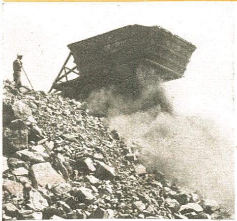
At the dumping place, the tractor driver pulls a lever and the body of the trailer slides back beyond the end of the floor
