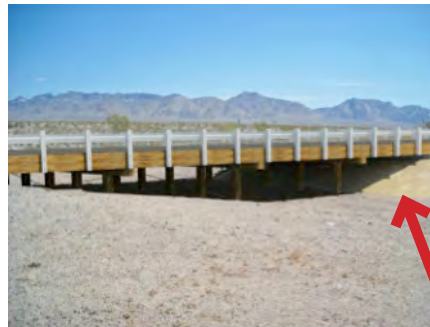
Figure 175 Simulation showing proposed 'W' shaped guardrail painted white (courtesy of San Bernardino County DPW); note post caps will also extend above the 'W' beam
