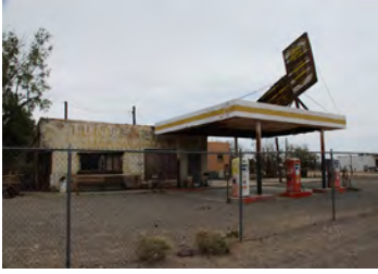
Figure 81 Former Whiting Brothers Garage, Newberry Springs
