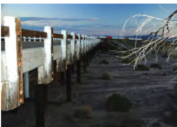
Figure 74 Timber trestle bridge at Avon Wash
