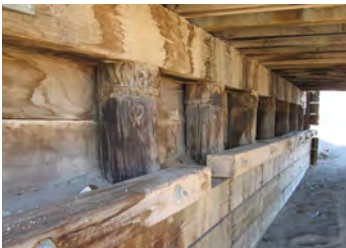
Figure 73 Underside view of existing timber bridge structure
