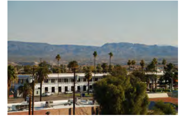
Figure 121 The restoration of El Garces in Needles presents an important opportunity to establish a gateway site for visitor information and interpretation
