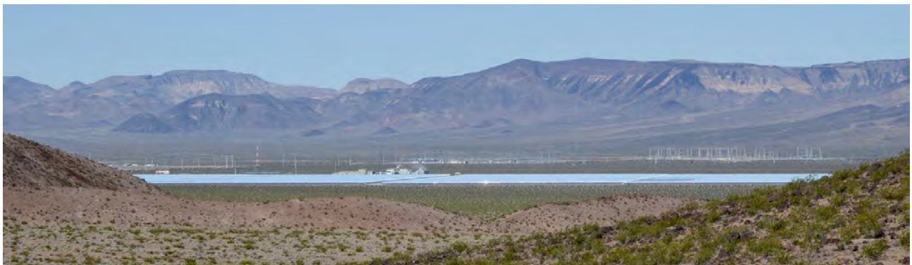
Figure 87 Photograph of Nevada Solar One near Boulder City, Nevada illustrating very high levels of visual contrast and the expansive scale of a utility scale solar facility. Credit: Robert Sullivan, Argonne National Laboratory.
