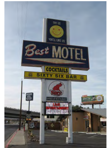
Figure 104 The Best Motel in Barstow is an example of a remodeled motel from the early 1960s. This was originally an Imperial 400 Motel which was designed with a distinctive “gull wing” roof at its lobby. The building has added exterior wall surfaces, windows and doors.
