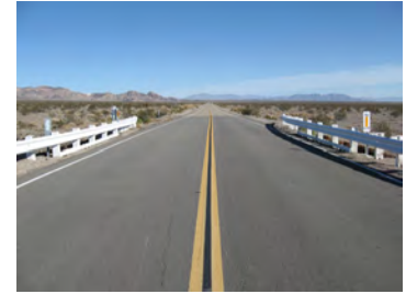
Figure 167 The recently reconstructed Amboy bridge maintains the white finish and uses a W-beam guardrail which has been reinforced with a double thickness for crash-worthiness.
