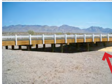
Figure 171 Existing Dola Bridge elevation (above) and two options for bridge abutment treatments (arrows): concrete (top right) and timber (bottom right). Simulations courtesy of San Bernardino County DPW; note post caps will extend above the 'W' beam which will be reinforced by joining two 'W' beams together to increase its strength without increasing the height and proportion of the railing.
