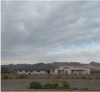
Figure 206 Adaptive re-use of the Amboy School complex could provide needed visitor services for attracting more niche groups to Historic Route 66.
