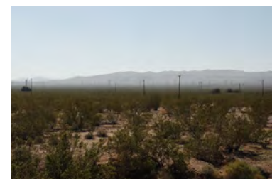
Figure 82 Existing high voltage electric transmission lines east of Daggett
