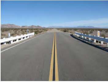
Figure 107 Historic Route 66 east of Amboy
