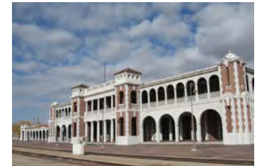
Figure 122 The Barstow Visitor Center is already located at the Harvey House
