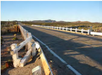
Figure 72 Existing timber bridge rail with 'C' shaped metal approach rail
