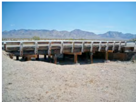
Figure 171 Existing Dola Bridge elevation (above) and two options for bridge abutment treatments (arrows): concrete (top right) and timber (bottom right). Simulations courtesy of San Bernardino County DPW; note post caps will extend above the 'W' beam which will be reinforced by joining two 'W' beams together to increase its strength without increasing the height and proportion of the railing.
