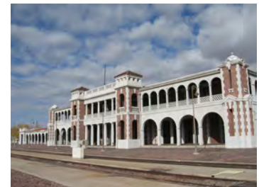
Figure 44 The restored Harvey House in 2013
