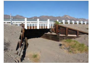
Figure 75 View of bridge rail and abutment walls at Amboy bridge
