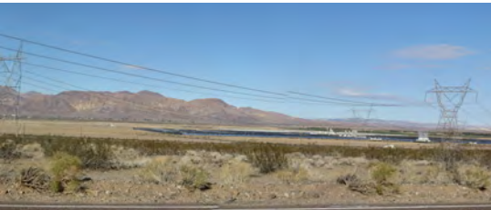
Figure 64 Existing solar project between Daggett and Newberry Springs
