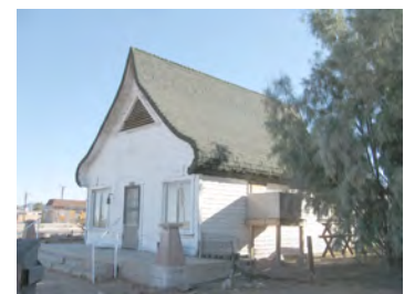
Figure 141 Former cafe near Daggett
