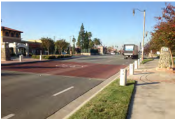
Figure 179 Pavement markers are combined with other elements in Rancho Cucamonga to improve visibility and enhance the streetscape
